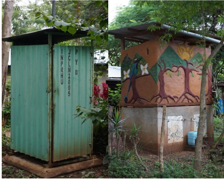
Figures 3a & 3b. An ecological dry latrine (right) developed by Grupo Fénix designed to replace the pit latrines (left) in the community that are beginning to threaten groundwater, one of many challenges associated with water the community is confronting. Photo credit: Michael Smith
